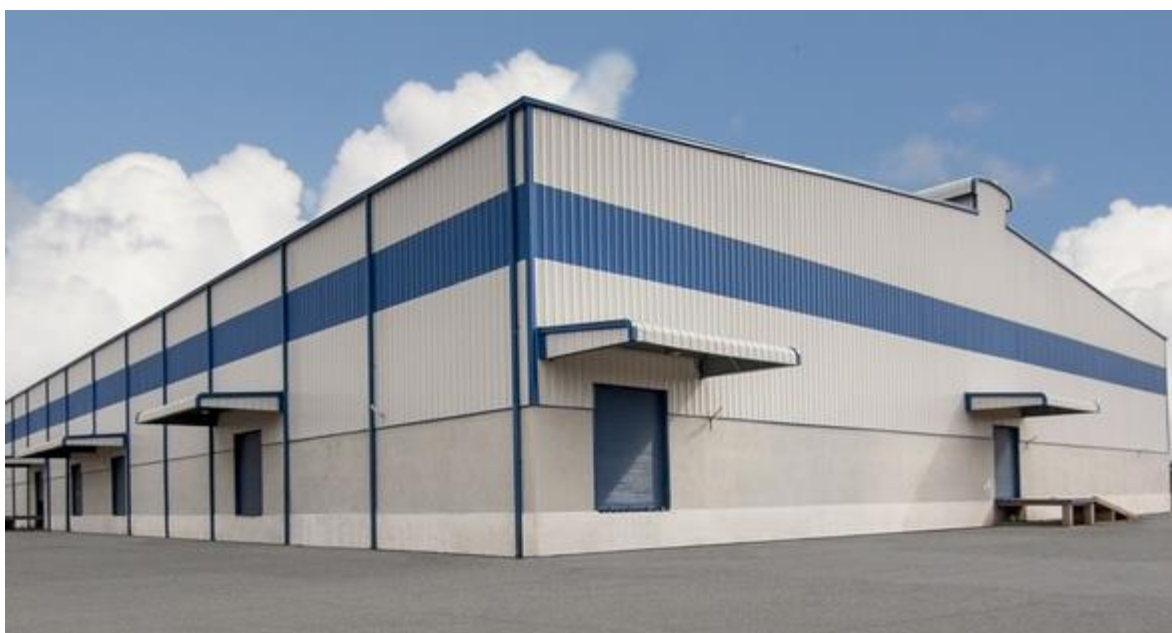
Figura 3-18 Nave industrial Shipsporter S.A. [59]
