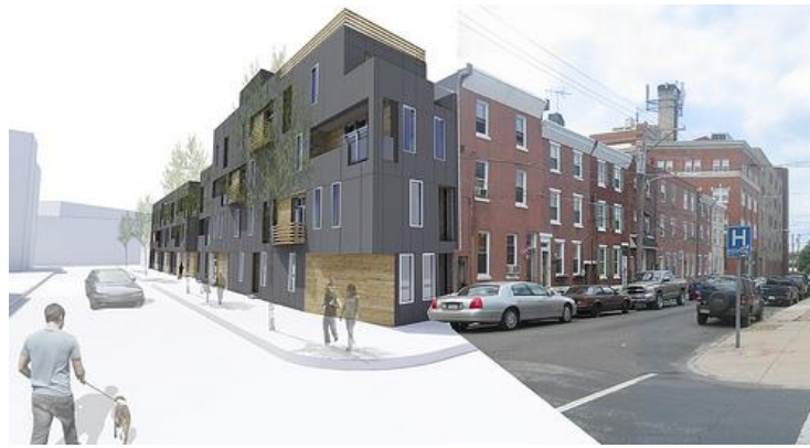
Figura 3-13 100K House Project (tomada de [11])
