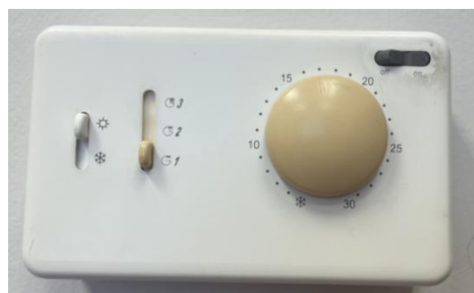
Figura 3-8 Panel de control regulable del fancoil
