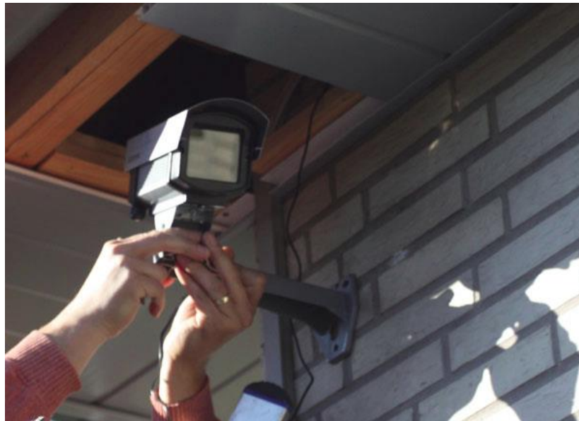
Figure 5-1 Raspberry Pi inside a CCTV casing (taken from [70])
